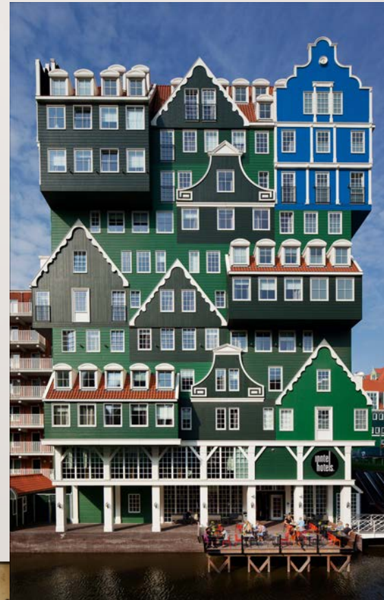
Inn Hotel, WAM architecten, (2010)
