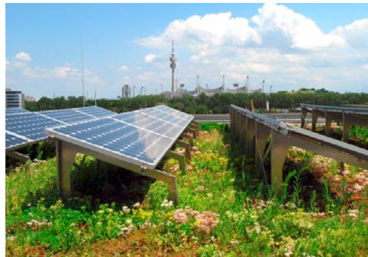
Slim energiedak in Rotterdam.
